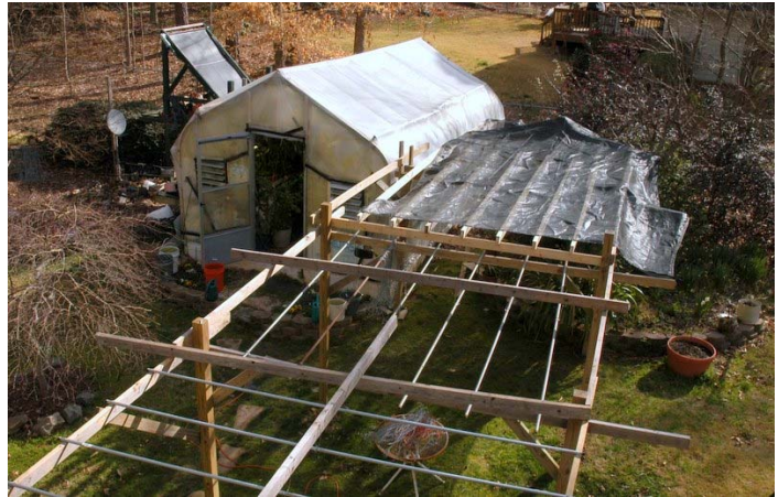
GREENHOUSE & SHADE STRUCTURE
